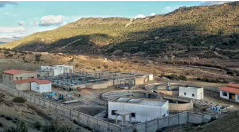
Estación depuradora de Arris en Wilaya de Batna, Argelia Arris water treatment plant in the province of Batna, Algeria
