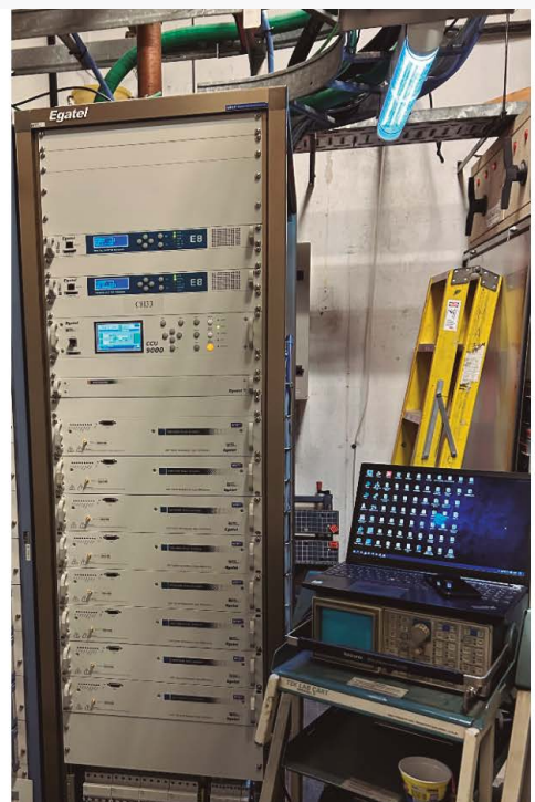
11.5KW ISDBT transmitter installed in the iconic Alas Building in Buenos Aires (Argentina).
