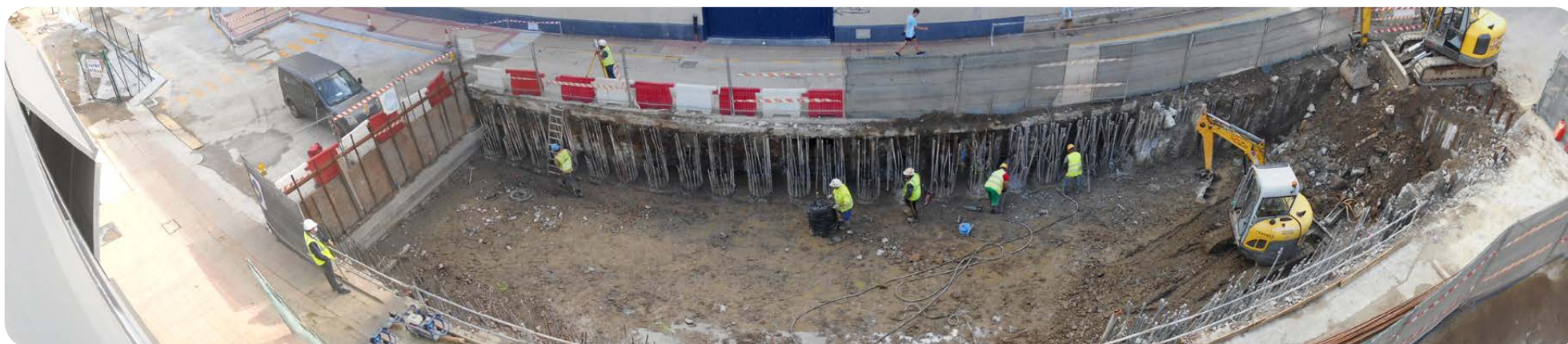
Preparation of the ramp for the execution of the false tunnel in the Galindo storm tank project, between Barakaldo and Sestao (Spain).
