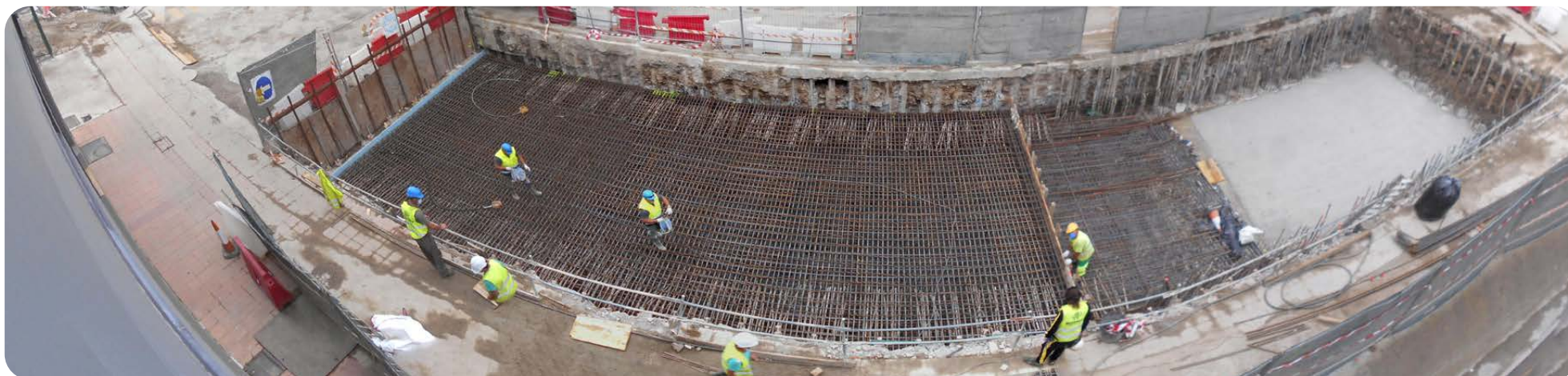
Construction of the slab over the execution area of the cut-and-cover tunnel in the Galindo storm tank project, between Barakaldo and Sestao (Spain)
