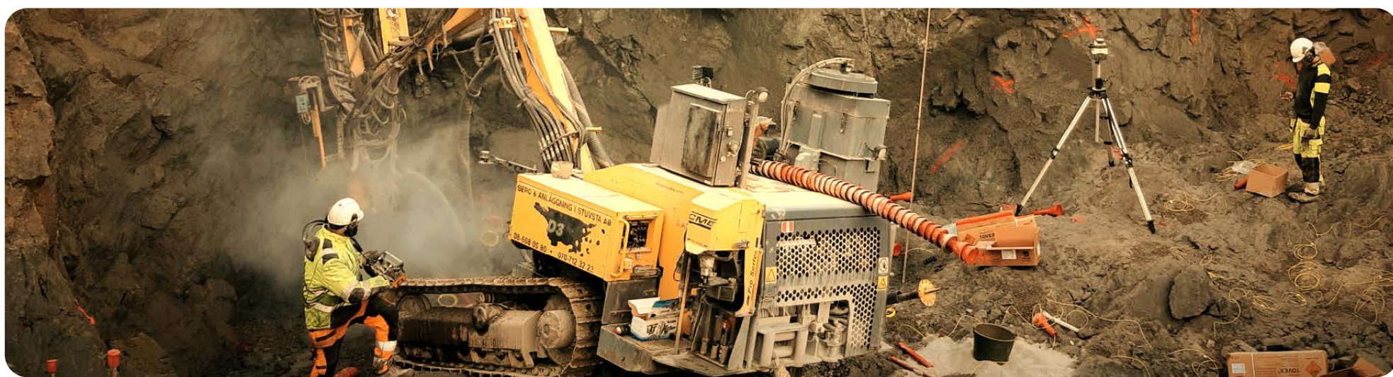
Drilling for the construction of the access tunnels to the E4 motorway, Skarholmen (Sweden)
