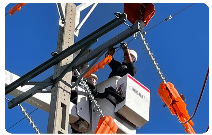
Installation of protections in medium voltage pylons, Salamanca (Spain)
