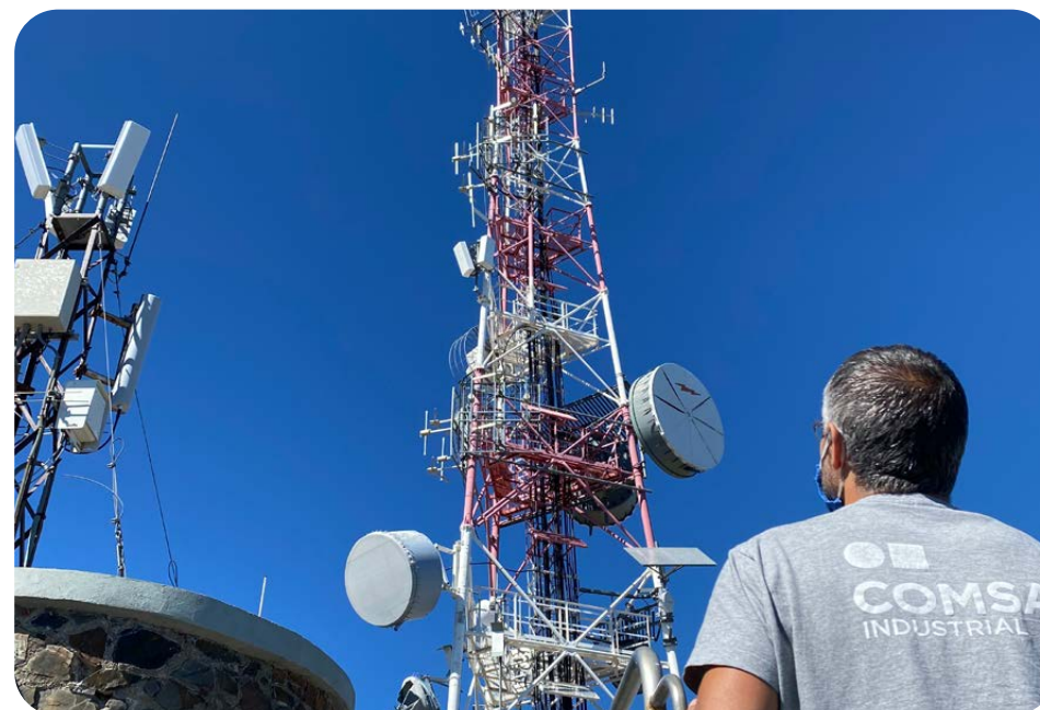
Corrective maintenance of FM broadcasting antennas, Pic de Carroi (Andorra)
