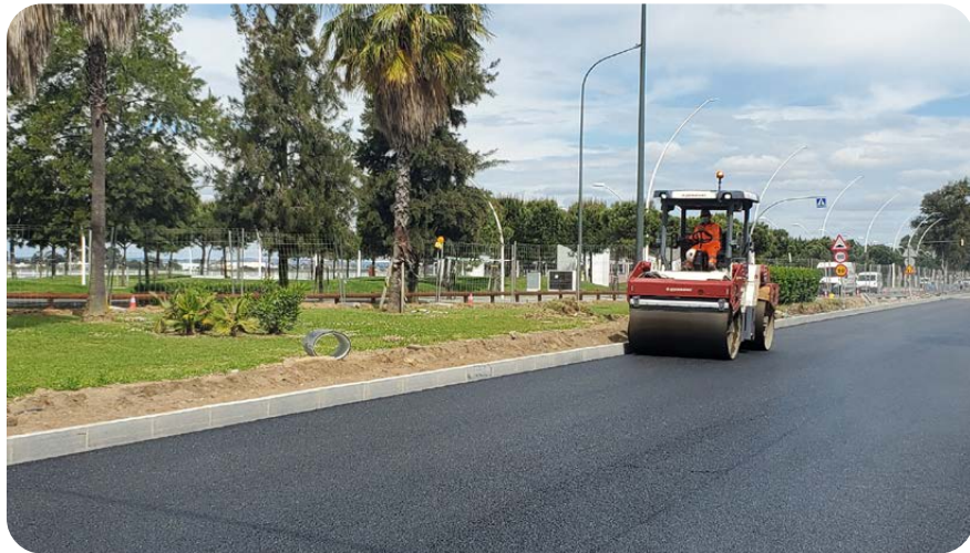
Anti-cracking road construction with tyre powder with high recycled rubber content, Huelva (Spain)
