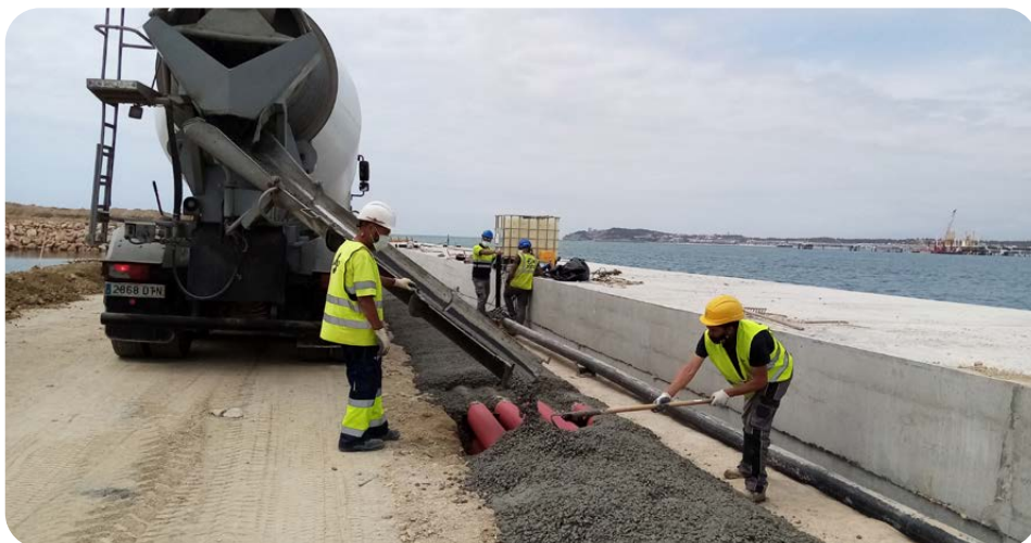
Concreting works in the new Baleares quay of the Port of Tarragona (Spain)
