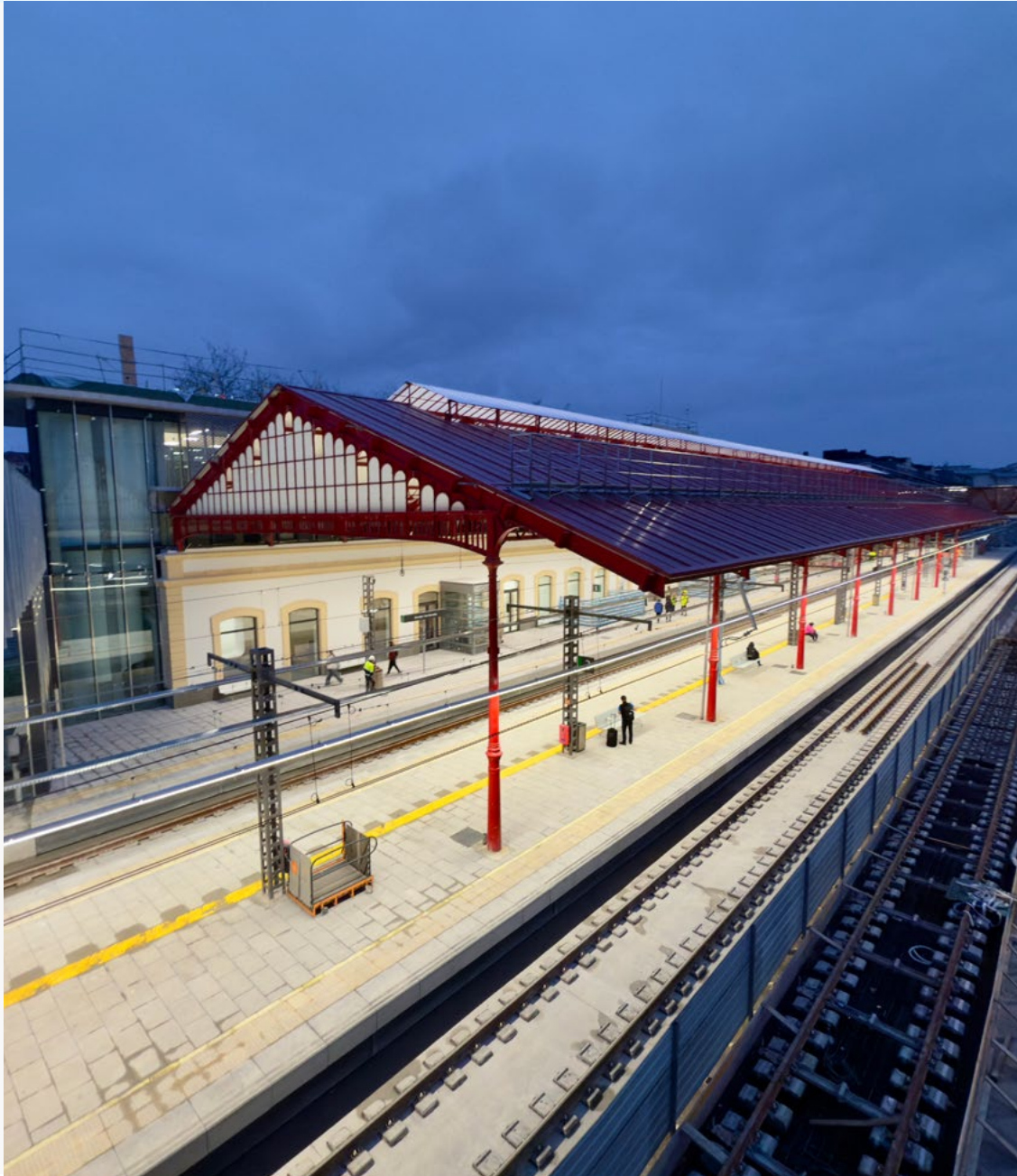
Renovation of Atotxa station, San Sebastián (Spain). ►
