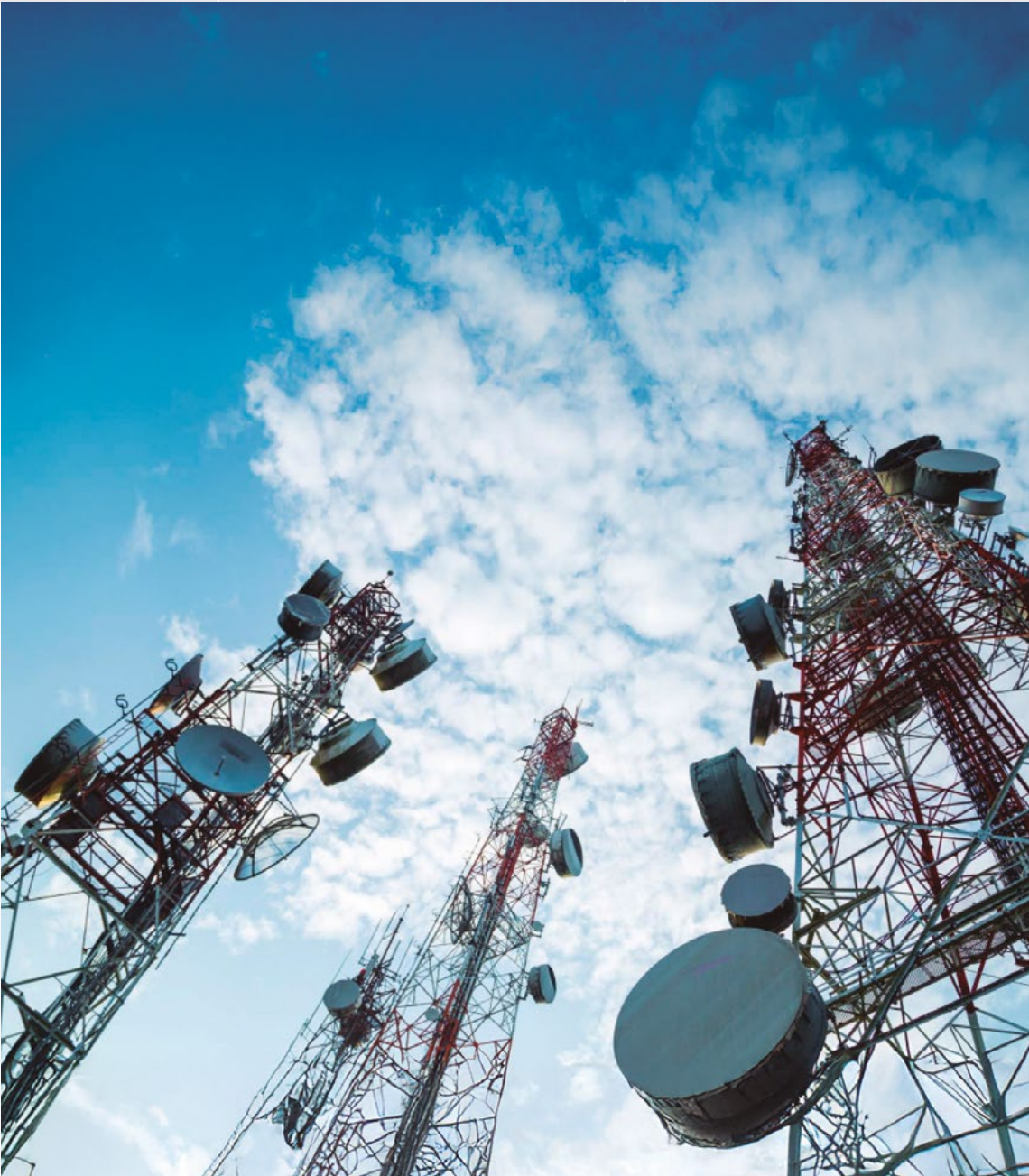
Maintenance and adaptation of the Canal de Isabel II, Madrid (Spain). communication towers. ▶
