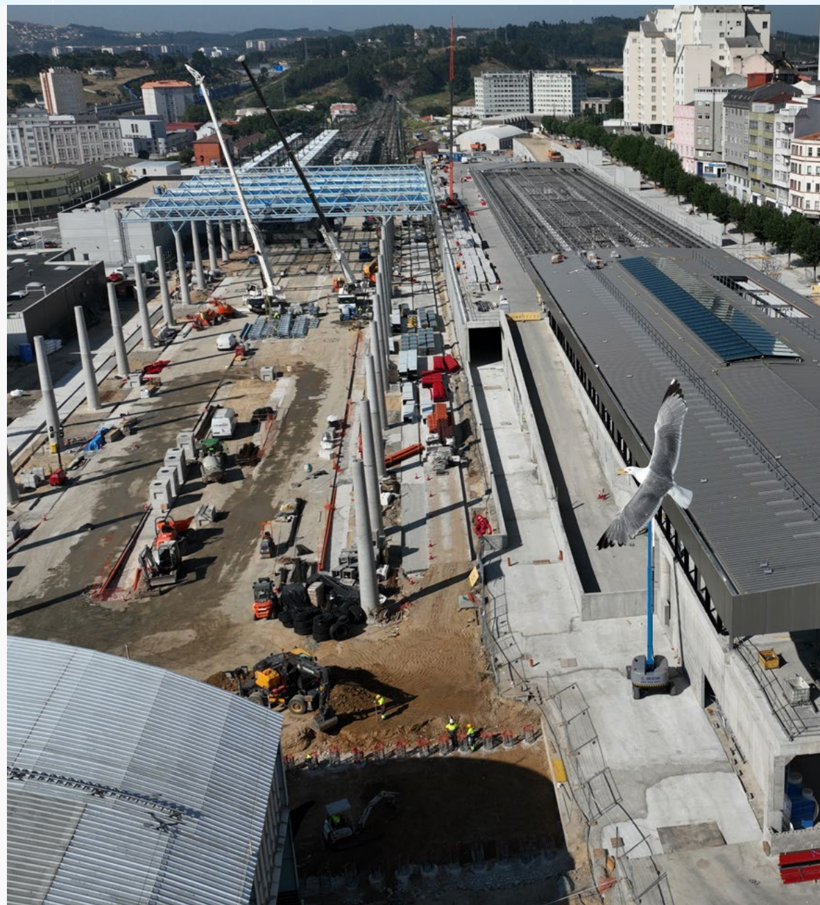
Construction of the new bus station in the Intermodal area, A Coruña (Spain). ►
