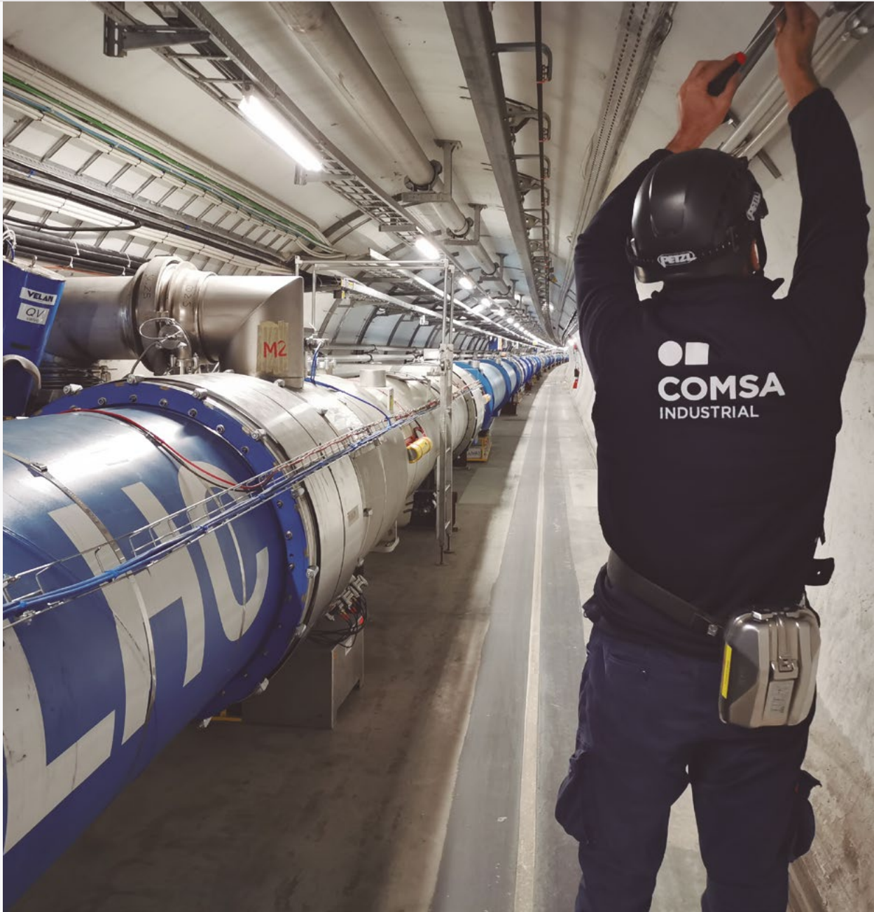
COMSA Industrial carries out renovation works of the electrical installations and networks and telecommunications support at the CERN headquarters, Preveessin and Meyrin (France and Switzerland).
