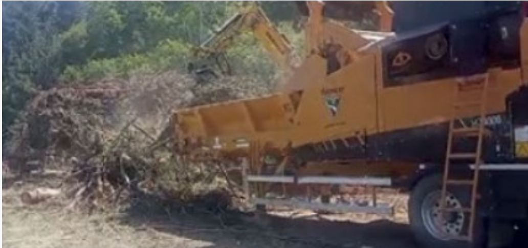
▲ Use of woody material from felling to improve the topsoil of the worksite, helping to retain water, improving aeration, and preventing erosion.
