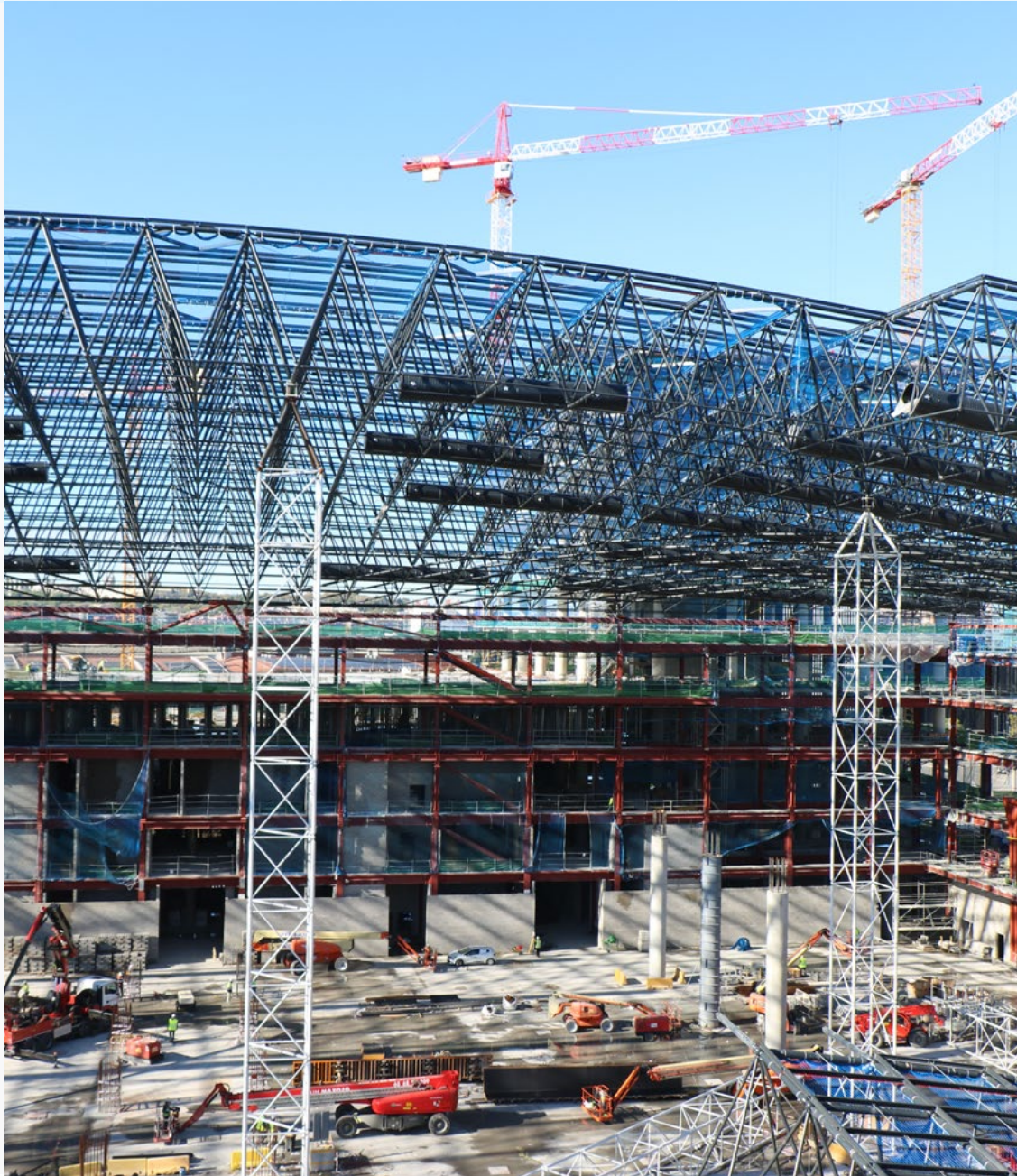
Construction of the new Hall Zero pavilion at Fira Barcelona (Spain). ►
