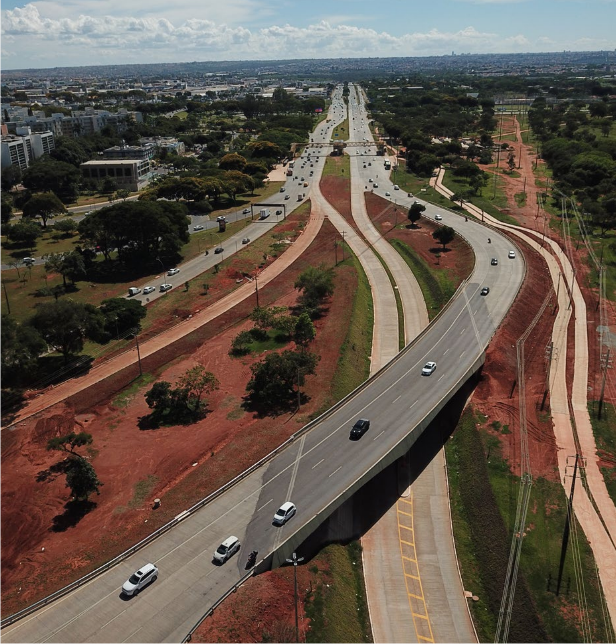
BRT works carried out on one of the main mobility axes of the area, Brasilia (Brazil). ▶
