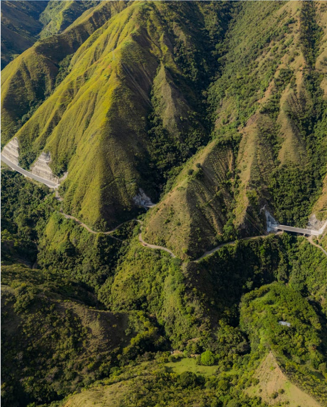
Installation of electromechanical, control, and radio communication equipment in the Guillermo Gaviria Echeverri Tunnel, known as the Toyo Tunnel, one of the longest in the country (Colombia). ▶
