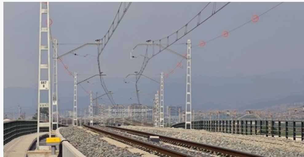
▲ Installation of 75 bird protection devices at the commuter access to Terminal T1 of Barcelona Airport (Spain).
