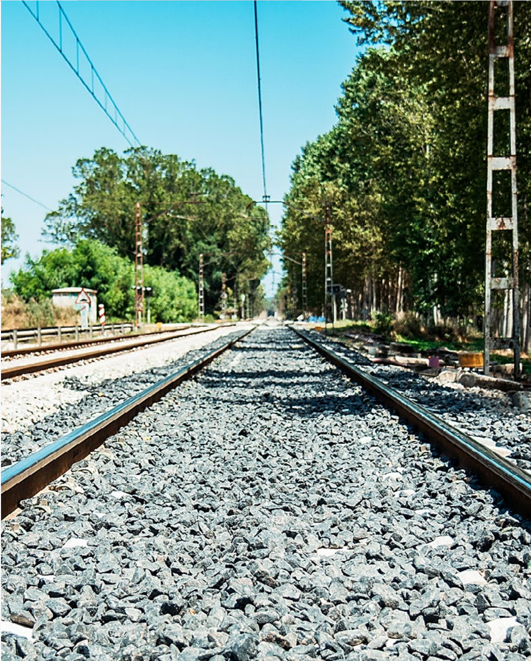
Tests conducted with NEOBALLAST® in a real environment. ►
