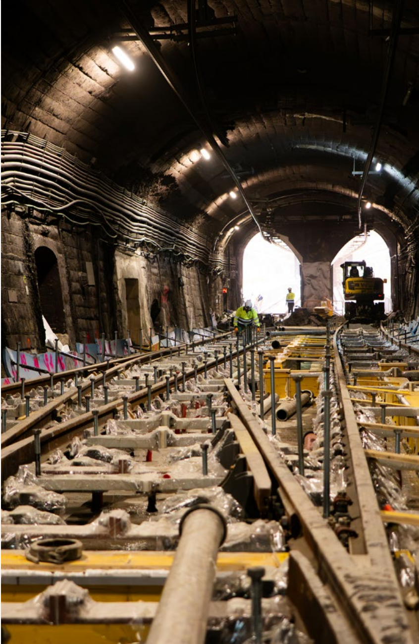
Renovation and automation of Line 6 of Metro Madrid (Spain). ►
