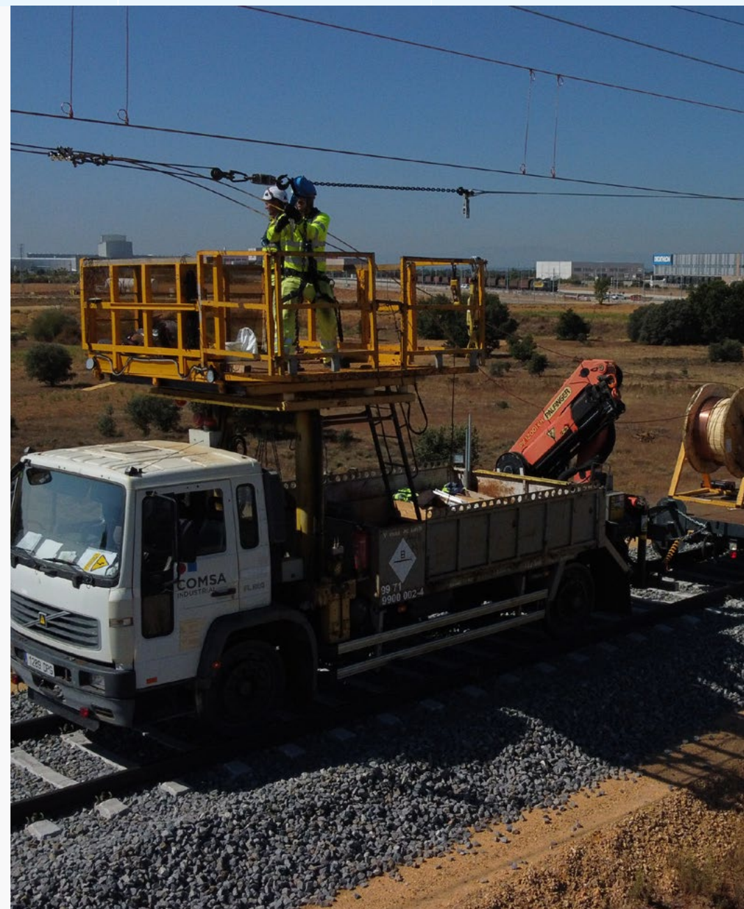
Laying and tensioning of contact wires in Villadangos, León (Spain). ►
