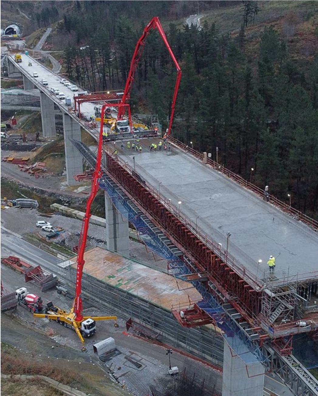
Completion of the Kortazar viaduct, within the construction works for the Basque high-speed line (Basque Y) (Spain).
