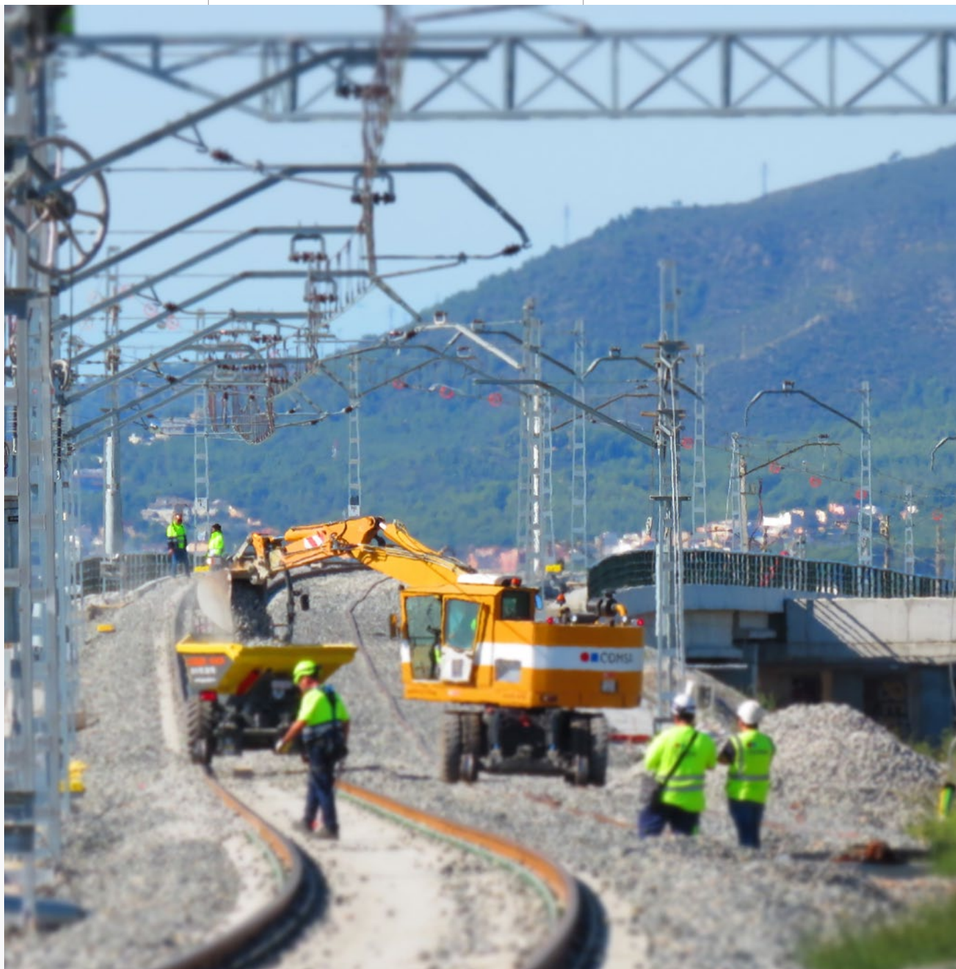
Terminal 1 access works at Barcelona-El Prat Airport, ► Barcelona (Spain).
