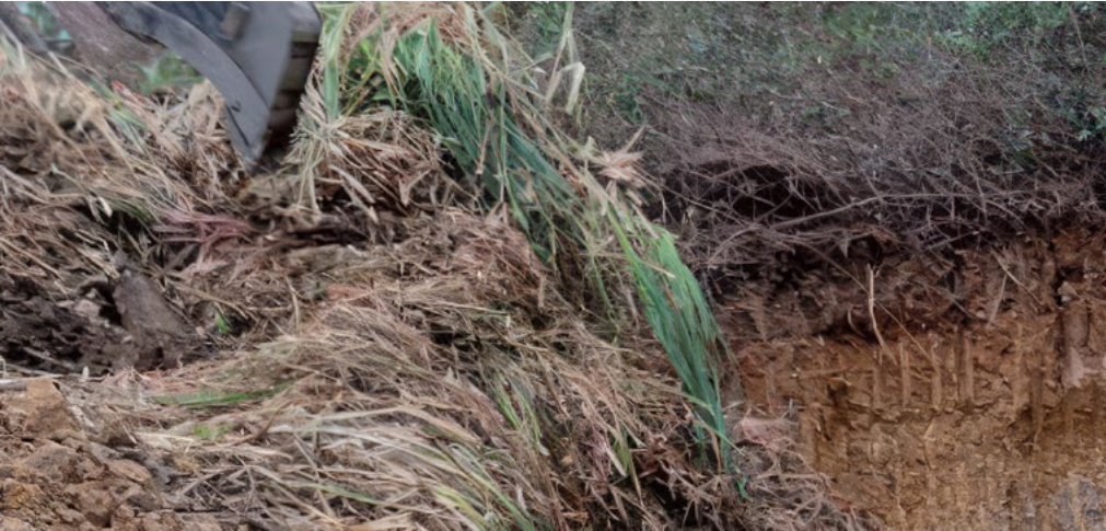
▲ Removal of the invasive species Cortaderia Sellonada on 2,274 m² to prevent its spread and improve the quality of the construction environment.
