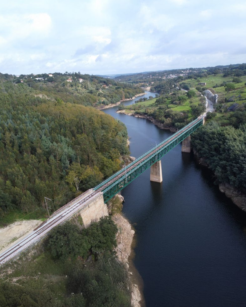
Works on one of the viaducts of the Beira Line in Portugal. ►
