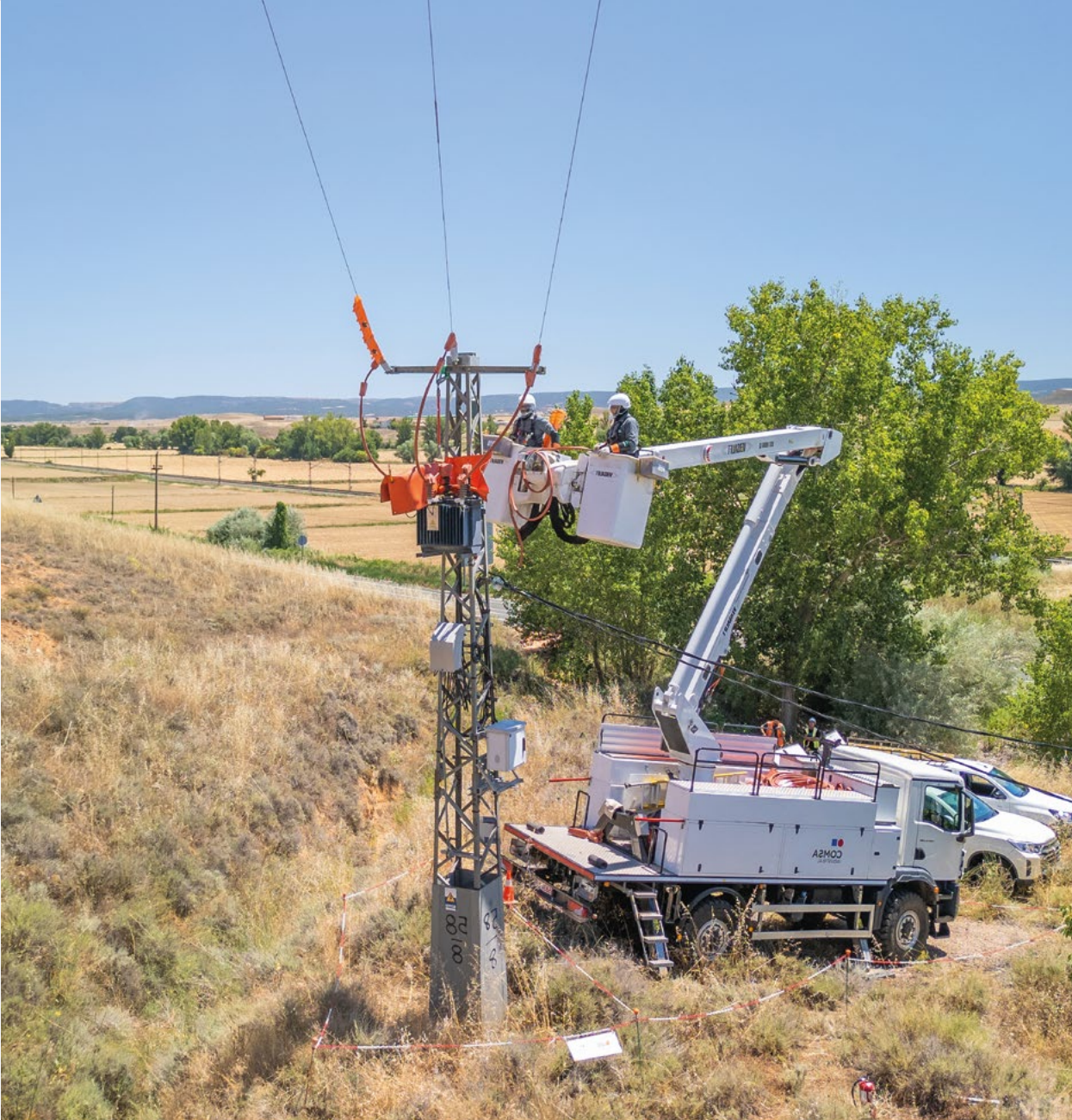
COMSA Industrial operation for UFD in the Arcos de Jalón, Soria area (Spain). ▶
