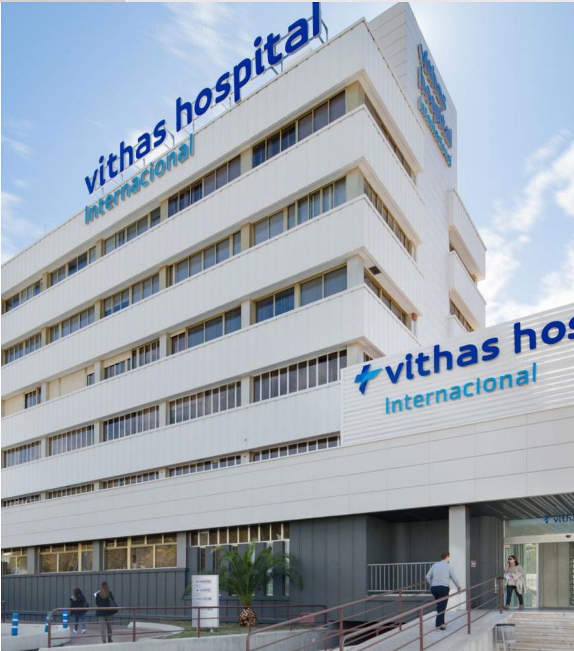
Specialized maintenance and renovation of hospital infrastructures. ►
