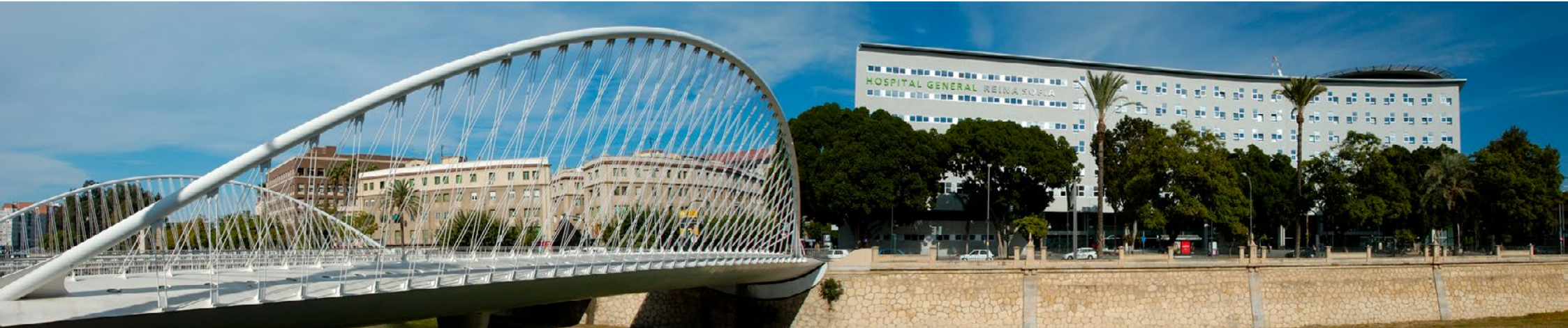
Maintenance carried out at Reina Sofía General Hospital, Murcia (Spain). ▼
