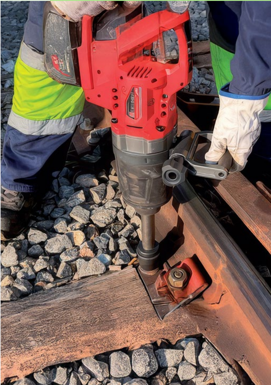
Electric impact nailers for maintenance work in the Barcelona Metro (Spain). ▶
