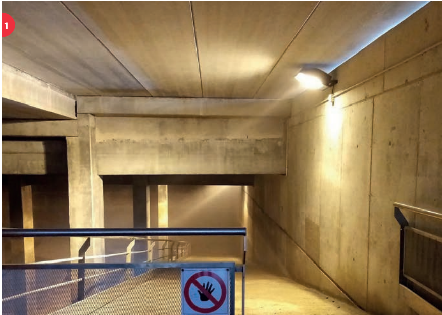
1 Interior del depósito de agua potable de Can Llong en Sabadell. Interior of the drinking water tank at Can Llong tank in Sabadell.
