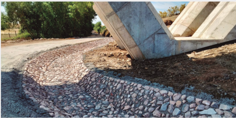
Landscape restoration of rivers with the reuse of 3,000 m 3 of rocks from the dismantling of railway tracks. New railway connection between Évora Norte and Elvas/Caia (Portugal).
