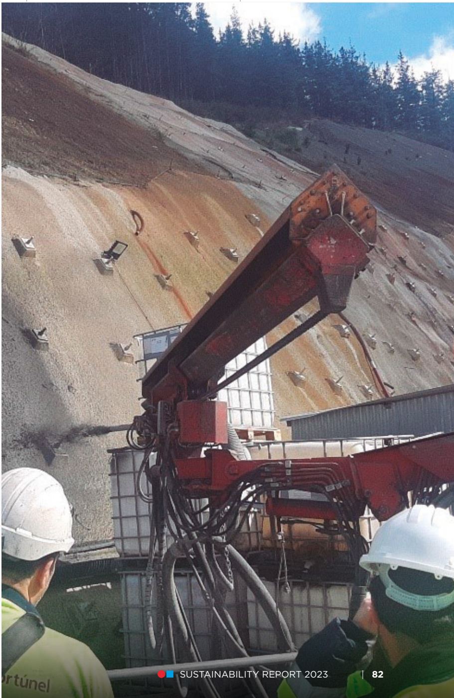
Spraying of recycled fibres from end-of-life tyres in the Elorrio tunnel (Bizkaia, Spain). ►
