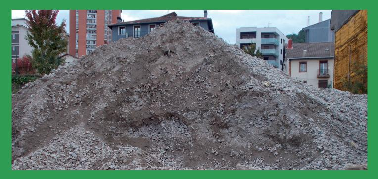
Reuse of recycled aggregates for the base of the foundation slab and external backfill of the basement walls of the building
