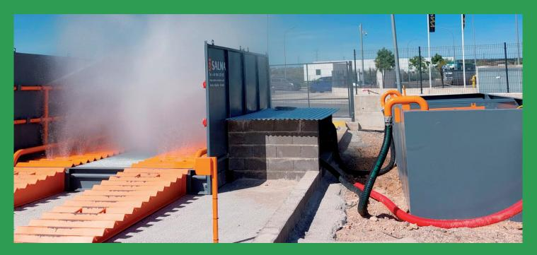
Wheel washing of construction site vehicles with closed water recirculation system
