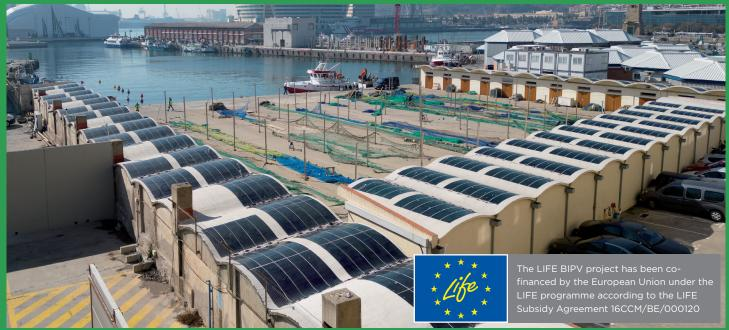
Flexible photovoltaic installation of 22.7kW on the huts of the Muelle de Pescadores
